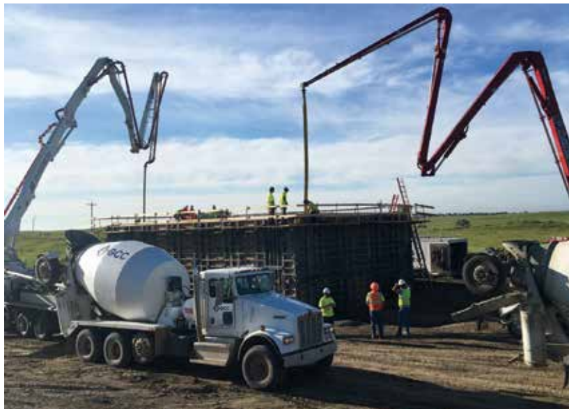
ABOVE: 410 cubic yards of cement went into the construction of a new 200,000 gallon reservoir east of Reservoir 5. This new reservoir will enable us to increase capacity during periods of peak demand.
