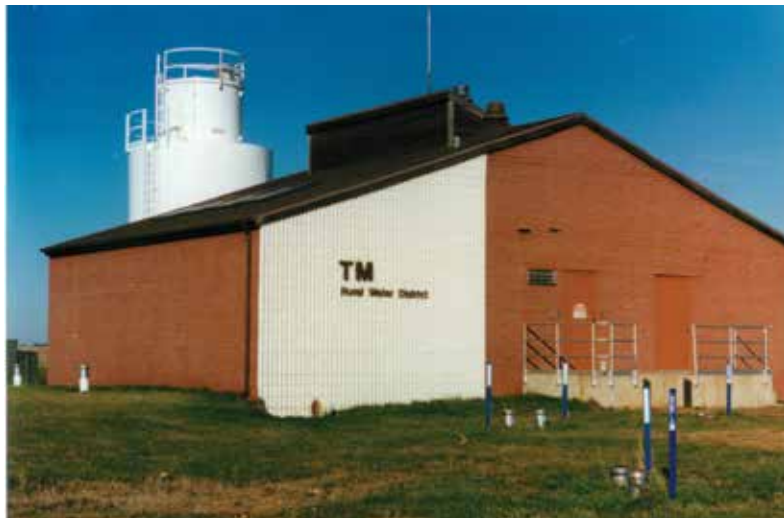
Original TM Water Treatment Plant
